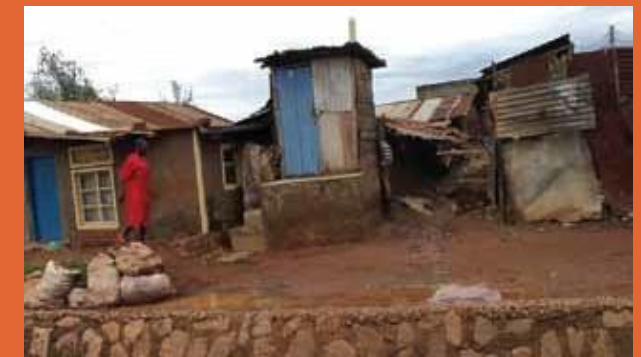
Elevated pit latrine in Kampala, Uganda
